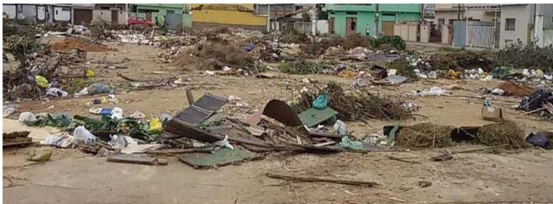
Figura 15: Descarte Irregular de RCC – Jockey Club
